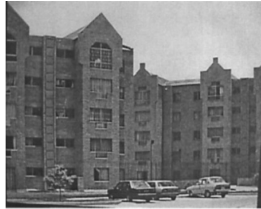
Fig. 2 Confined masonry in Colombia
