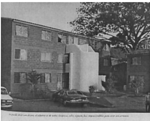
Fig. 1 Reinforced masonry in Mexico
