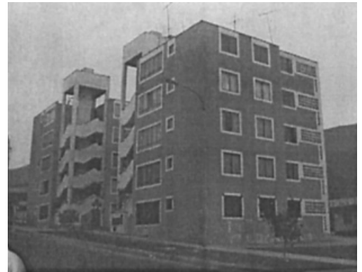
Fig. 3 Confined masonry in Perú
