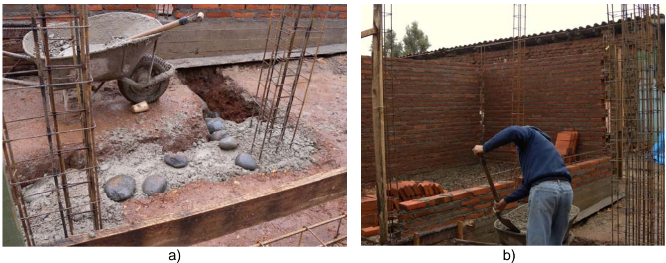
Figure 2. Key features of confined masonry construction: a) foundation construction (note tie-column reinforcement cages extending from the foundations), and b) wall construction.
