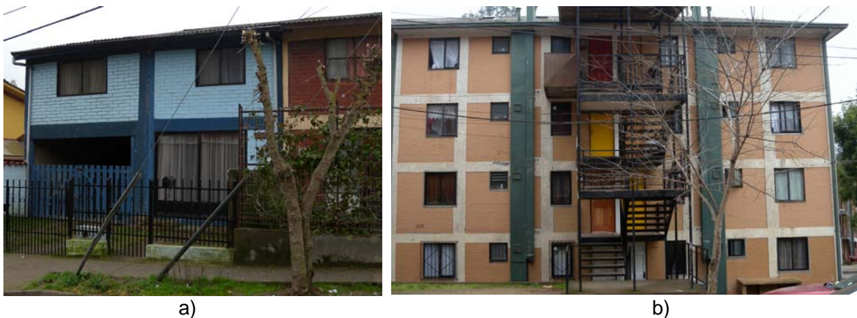
Figure 1. Typical confined masonry buildings in Chile: a) two-storey dwellings, and b) a four-storey apartment building.
