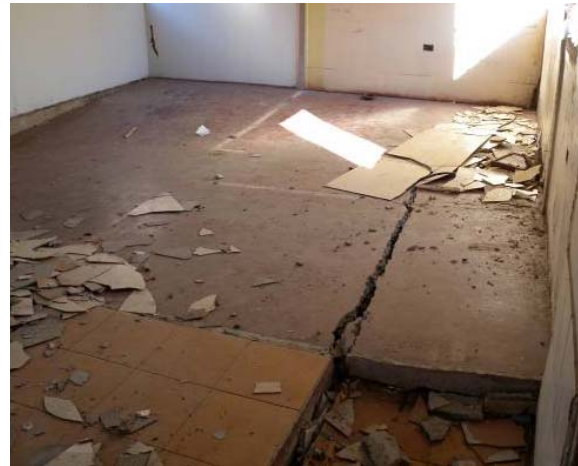
Figure 18. A building in Constitución experienced severe damage: a) extensive exterior damage in the building located closest to the creek located on the left side of the building, and b) extensive floor damage inside the building.
