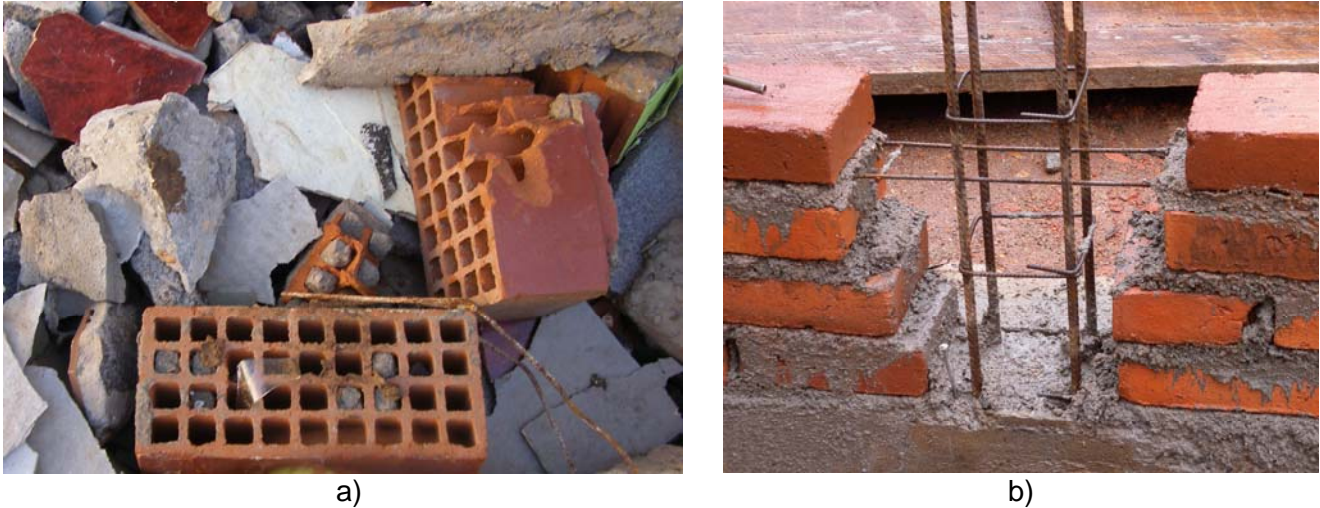
Figure 3. Confined masonry construction: a) a typical hollow clay unit, and b) a toothed wall-to-tie-column interface.
