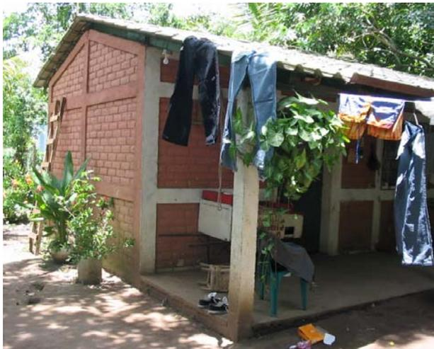
Figure 2. Representative mixto house used in reconstruction
