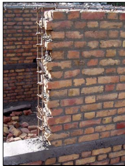
Fig. 10: Vertical reinforcements around openings
