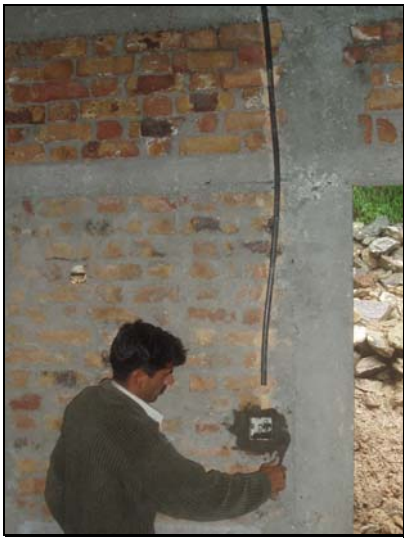
Fig. 15: No slits to be made in the masonry. Pipes can be hidden in the plaster, or left apparent
