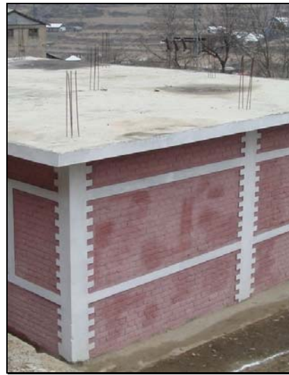
Fig. 16: Rebars on roof should be cast in lean concrete for protection
