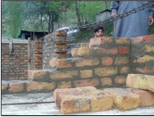
Fig. 7: Seismic band at lintel level
