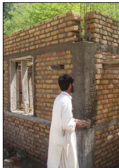
Fig. 6: Pouring concrete bit by bit
