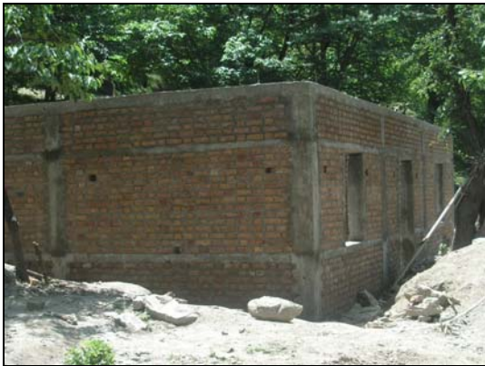
Fig. 3: Seismic bands at sill and lintel level
