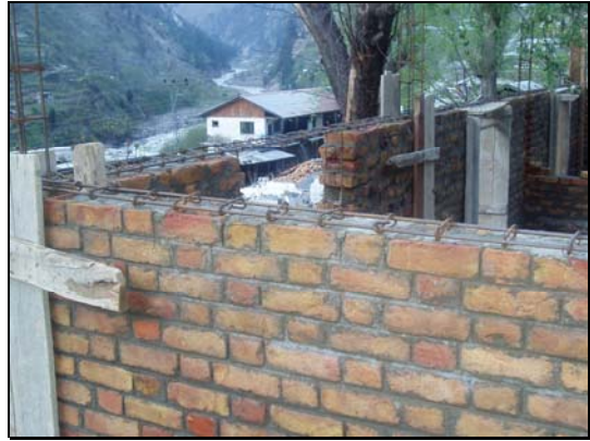
Fig. 8: Seismic band at lintel level
