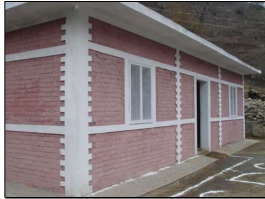
Fig. 2: Seismic reinforcements put in evidence through colour and mortar
