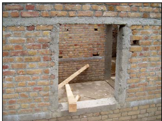
Fig. 12: Vertical bands around openings
