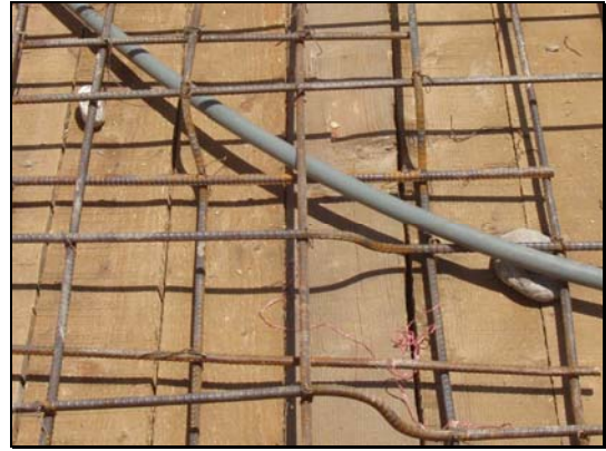
Fig. 14: Pebbles as spacers will not stay in place
