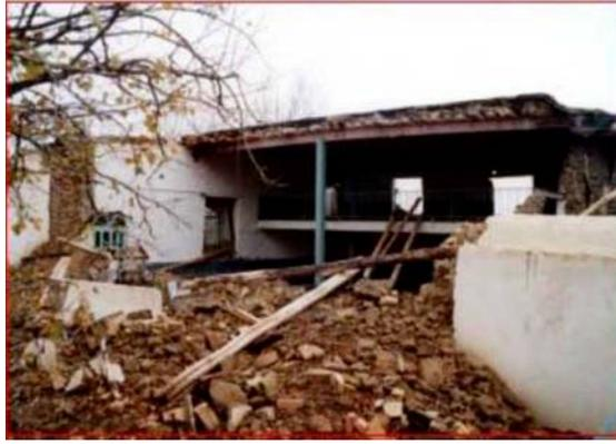
9. Roof failure in Abdoreh. Traditional post and beam system with no rigid joints between discrete elements cannot resist lateral force.
