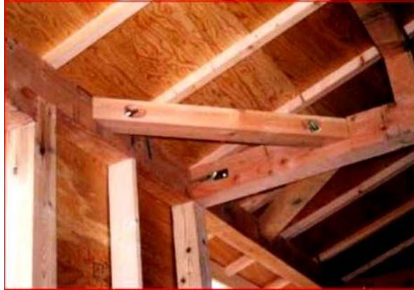
3. New school at the village of Chuzé donated by the Japanese government. The timber structure is designed and supervised by Japanese engineers. Note the metal joints tying the brace to the truss and the eave beam.
