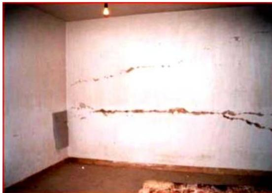
8. Classroom at Gerbanlu village, Hamadan province. Horizontal crack in non-load bearing partition caused by lateral forces of the earthquake for which it was not designed.
