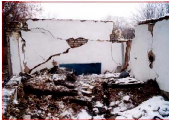
4. Ruined classroom at destroyed village of Changorreh in the province of Qasvin. The school was built in 1970 of thick unreinforced brick walls carrying a heavy mud roof supported on timber joists.
