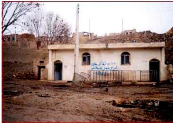
11. The public bath building is the only standing structure at the destroyed village of Abdoreh. It has several cross- and longitudinal- walls, which act as rigid diaphragms and make the whole structure behave like a box system.
