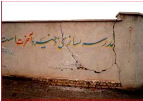
7. Hisar Wali 'Asr school in province of Qasvin. Cracks caused by Sliding shear in long boundary brick wall built without expansion joints.
