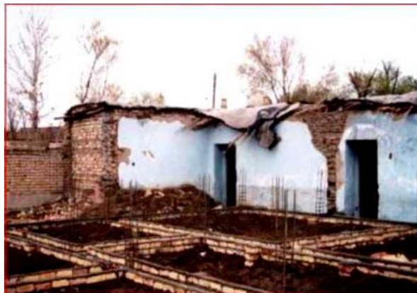
2. New school on the site of the destroyed elementary school in the village of Farsajin. Tie columns anchored to the reinforcement of the foundations and, eventually, to the ring beam confine the masonry and provide lateral resistance to walls. Note heavy walls and untied roof of collapsed school.
