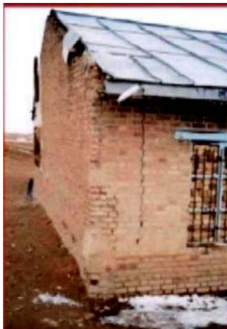
5. School building at Dornian village in Hamadan province. Built of unreinforced walls, hence the failure under vertical shear force. The lightweight roof saved the building from total collapse.
