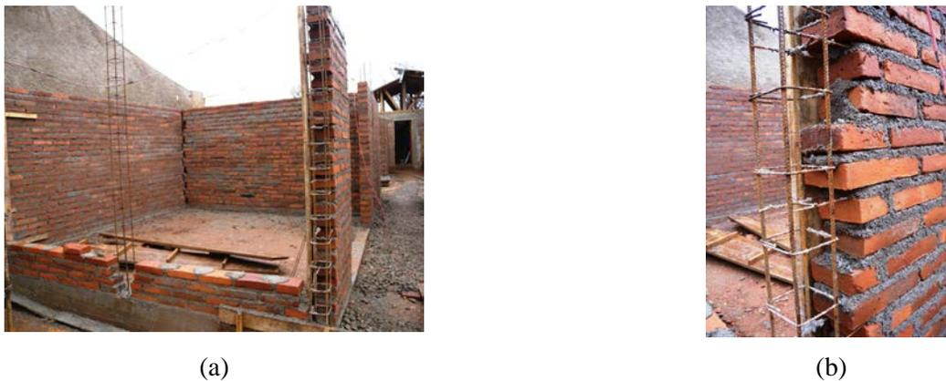
Fig. 2 – Confined masonry construction: (a) Masonry wall is built first and (b) a toothed wall-to-tie-column interface
