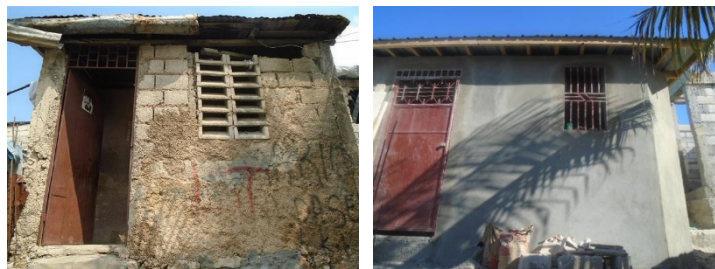
Fig. 4: A home in Port-au-Prince before (left) and after (right) a seismic retrofit
