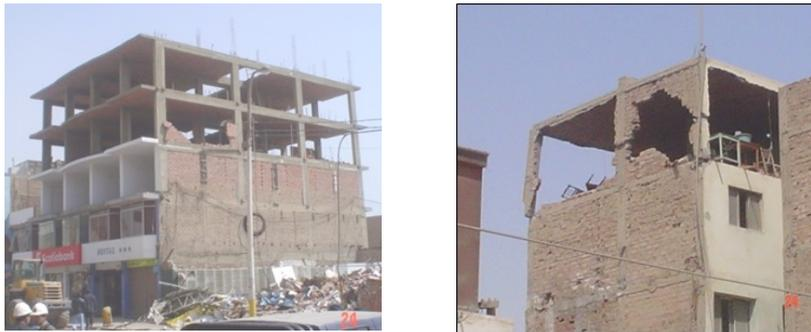
Fig. 11 – The 2007 Pisco earthquake revealed incorrect construction sequence in confined masonry
