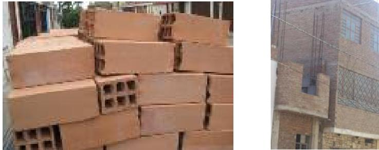
Fig. 10 – Hollow bricks with horizontal holes used informally in structural walls
