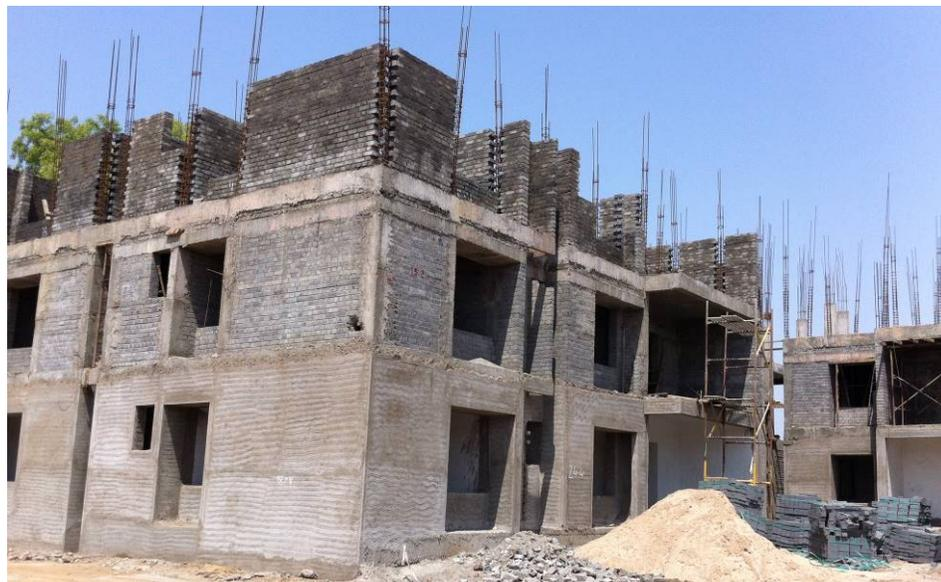
Fig. 1 – A confined masonry building under construction at the IIT Gandhinagar campus, India (Photo: S. Brzev)
